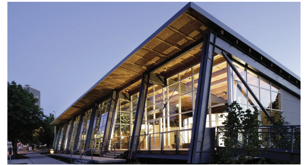
South Lake Union Discovery Center, Seattle, WA, Miller Hull Partnership
