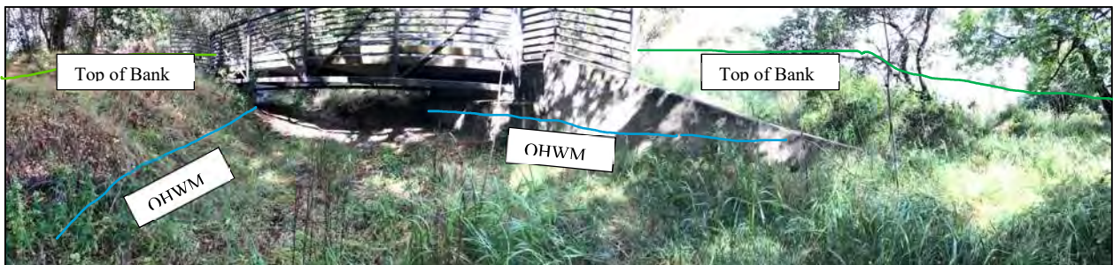
Photo 6. OHWM shown on the wingwall and channel bank.
