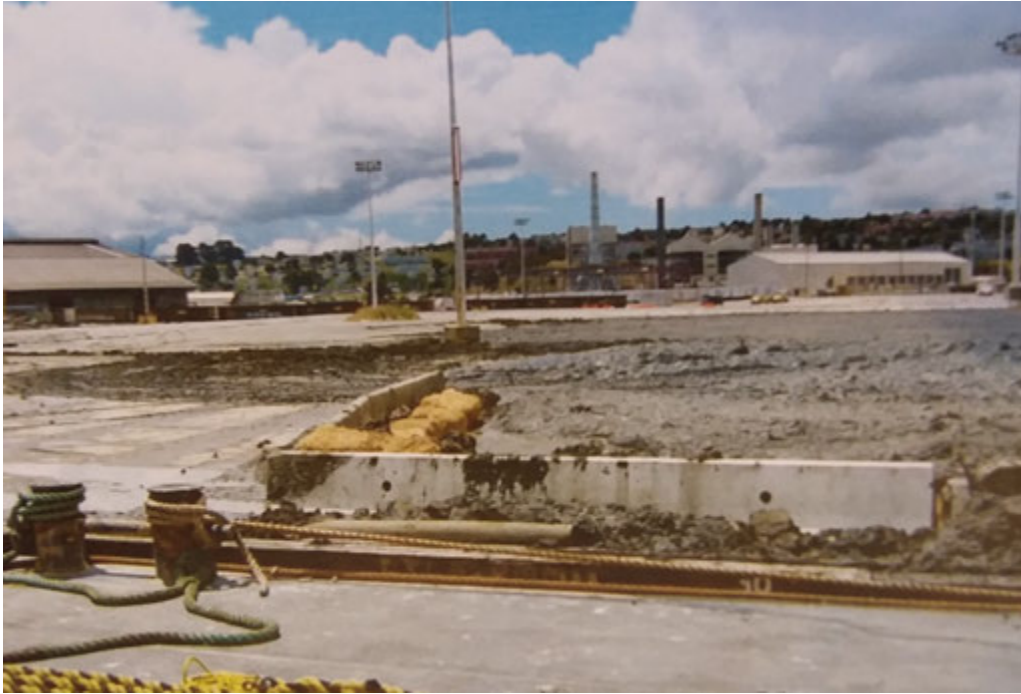
Figure 6-3 Contained Dewatering (Mechanical Dredging)
