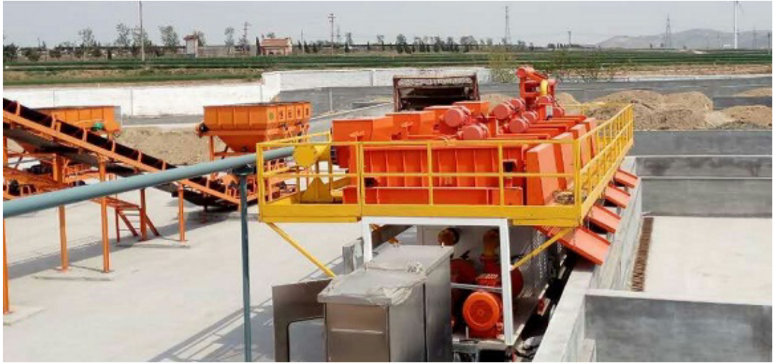
Figure 6-6 Rapid Dewatering System
