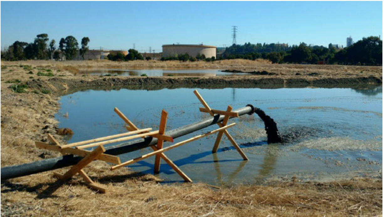
Figure 6-4 Settling Pond Dewatering (Hydraulic Dredging)
