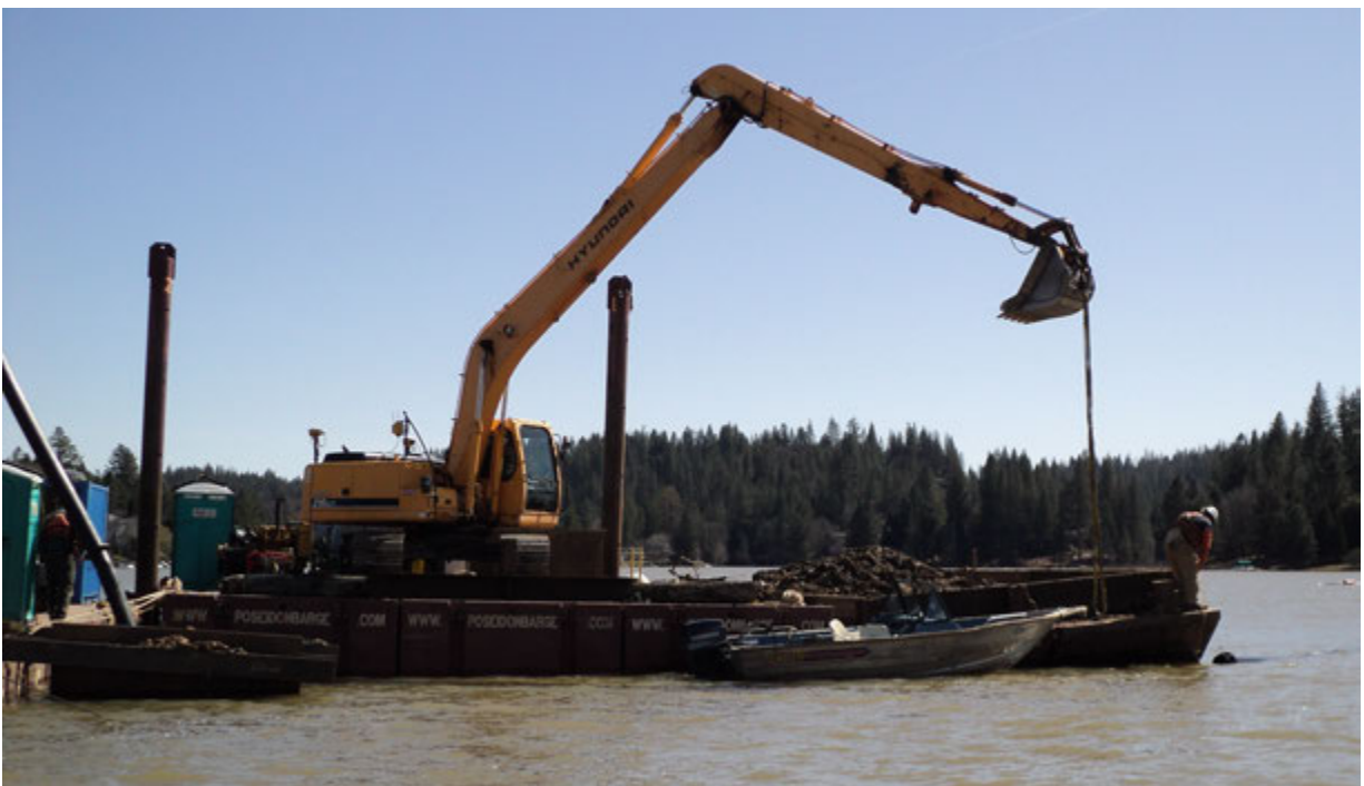
Figure 6-2 Small Mechanical Dredge Equipment
