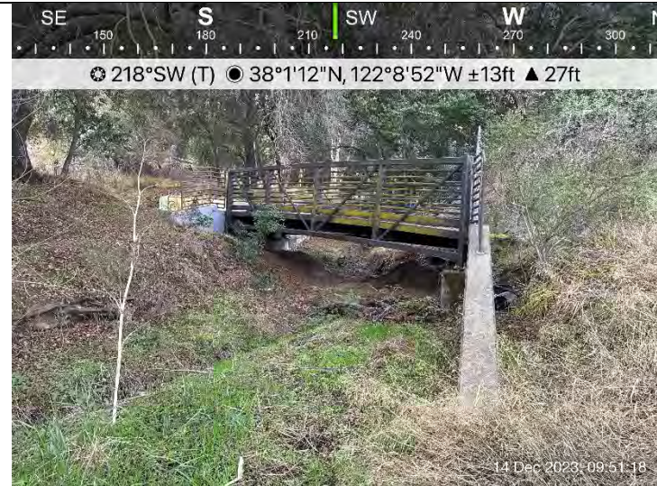
Photo 6. Pedestrian bridge crossing the unnamed channel occurring along the alignment.
