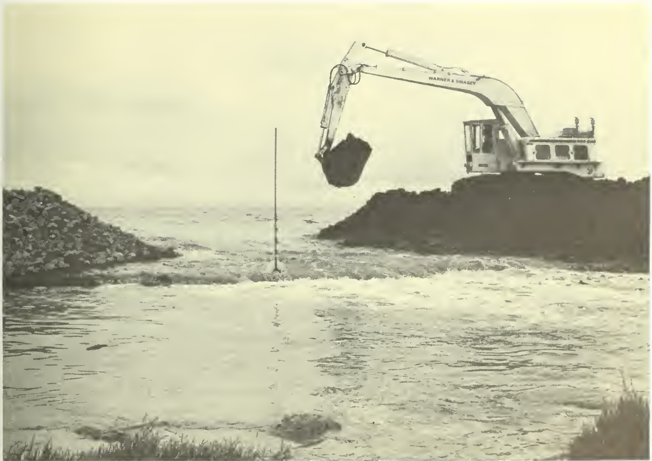
Hayward Regional Shoreline in the Making: In 1980 an outer dyke was breached and Bay waters flowed into a 200-acre area bringing renewed life and habitat for aquatic based creatures. Trails and boardwalks allow visitors to explore the rich shoreline environment, which is intended to remain natural.
