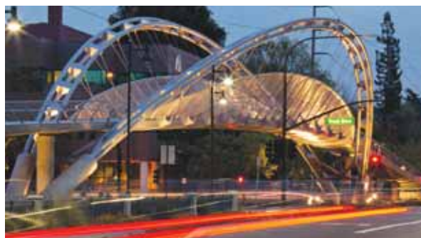
Robert I. Schroder Overcrossing Iron Horse Regional Trail, Pleasant Hill, CA
