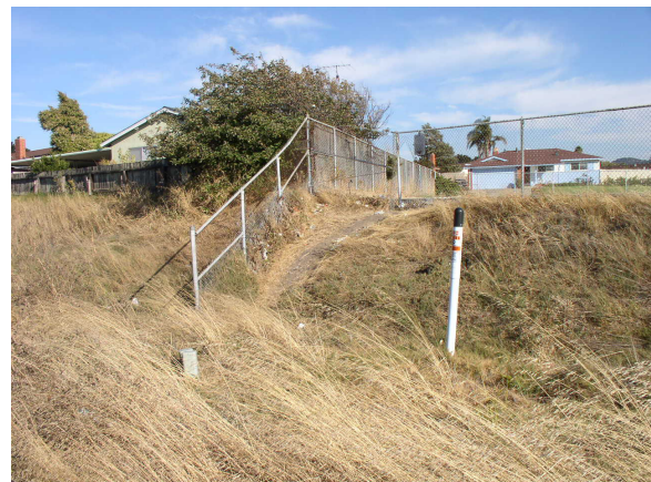
User defined pathways from adjacent properties show a clear pattern of trespassing. This photo illustrates a cut fence and worn trail leading from the Sea View School parking area into the UPRR ROW.
