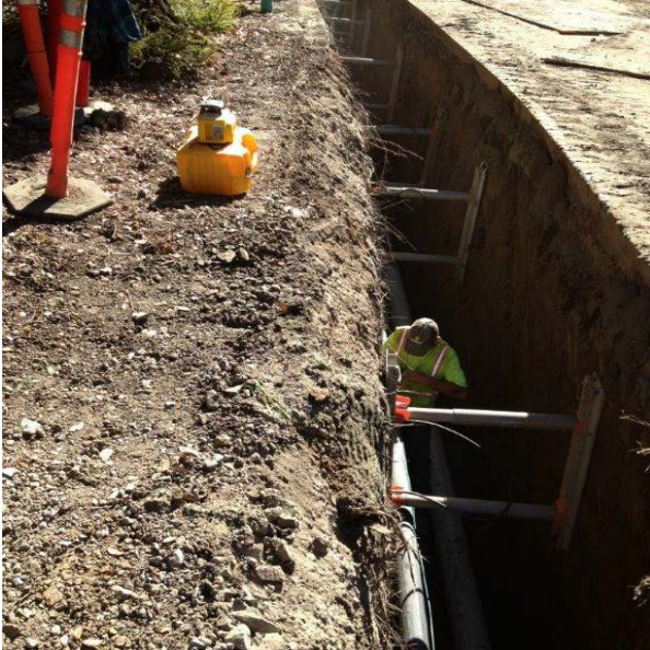
Top two photos is work in progress
