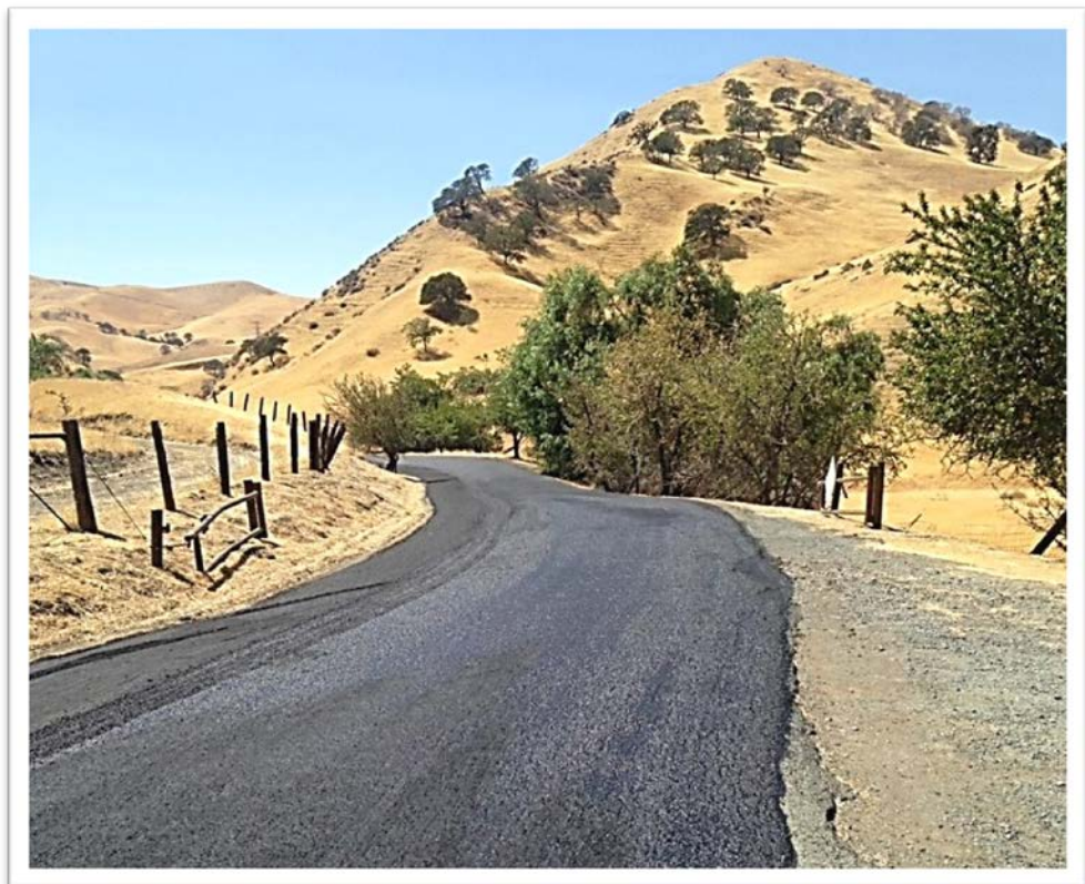
The photo above is the finished product.
