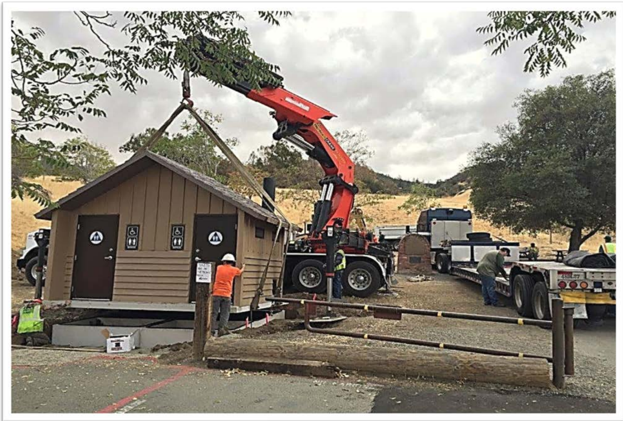
Installation of the CXT restrooms at Black Diamond.
