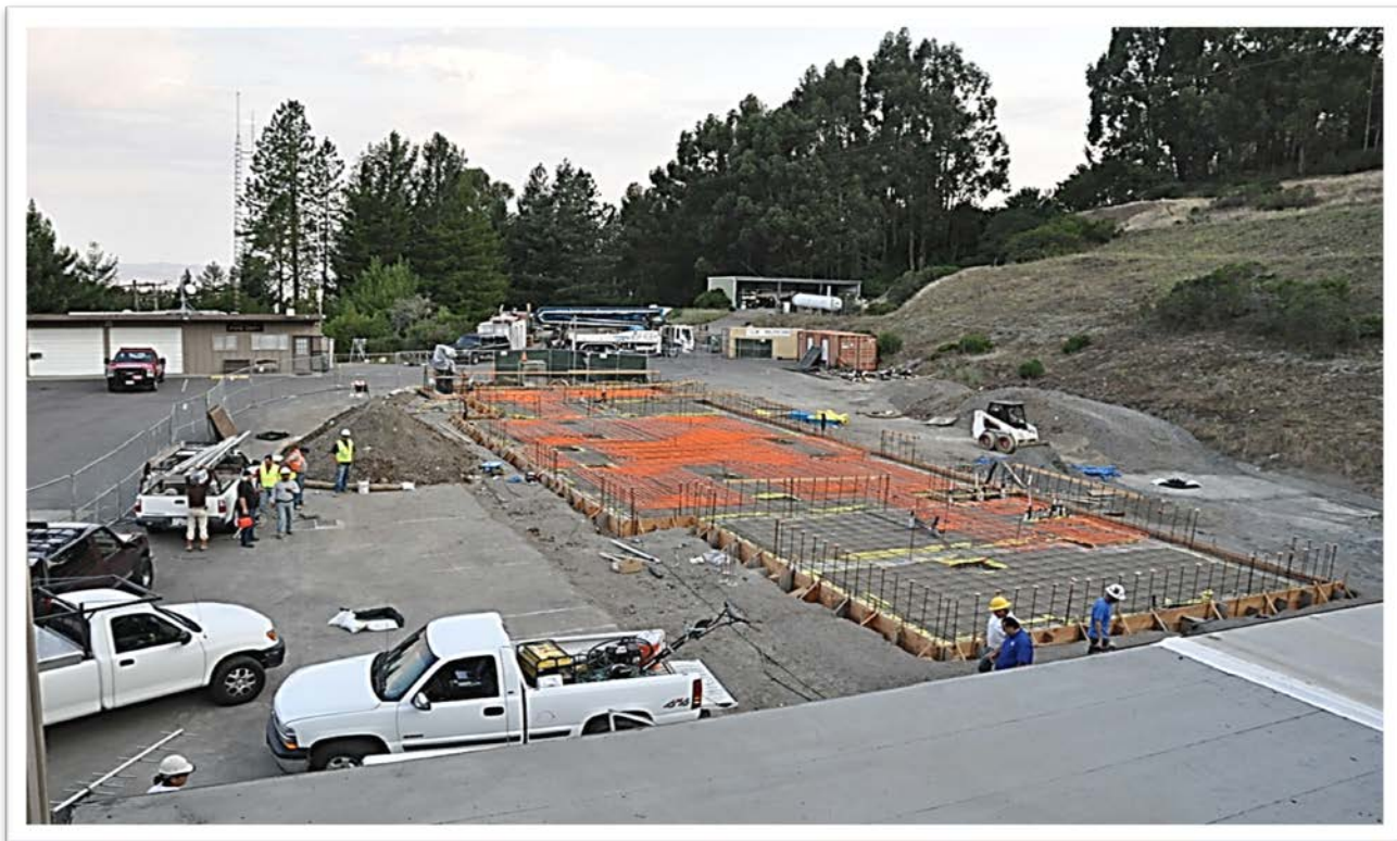
Installation of utilities under the slab.
