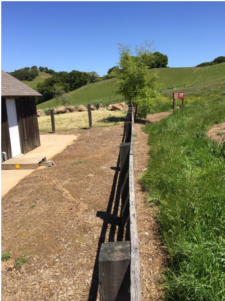
Figure 3. Typical integrated vegetation management in drier parks: Rough mowing around structures with a wider band of herbicide treatment to keep vegetation off wood fencing
