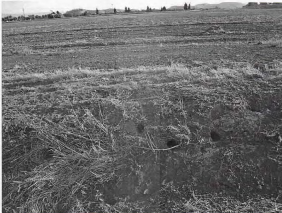
Photo 4: Burrows along berm
