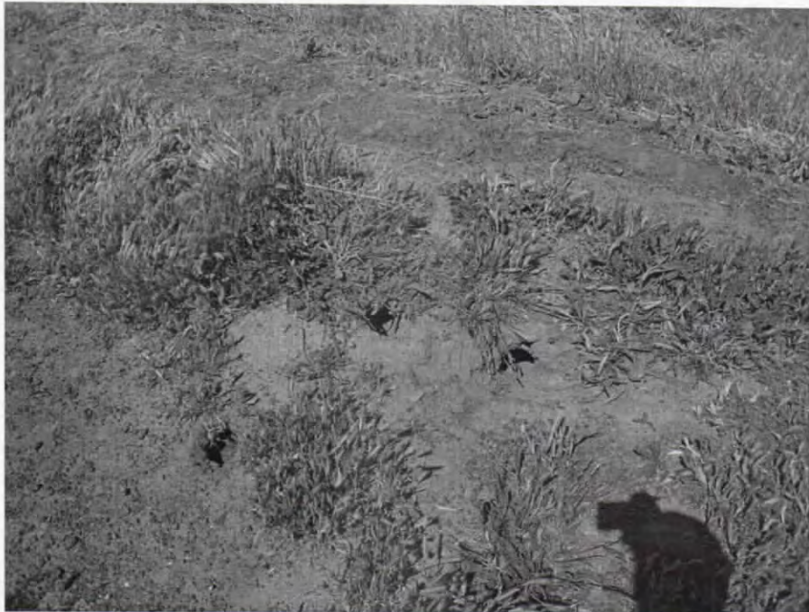
Photo 4: Burrows along berm
