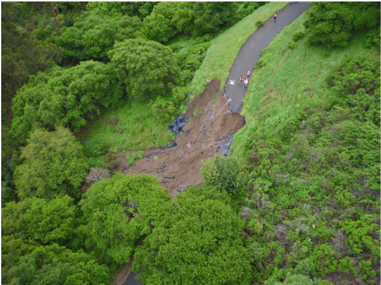
Aerial view of landslide at Gelston Road.
