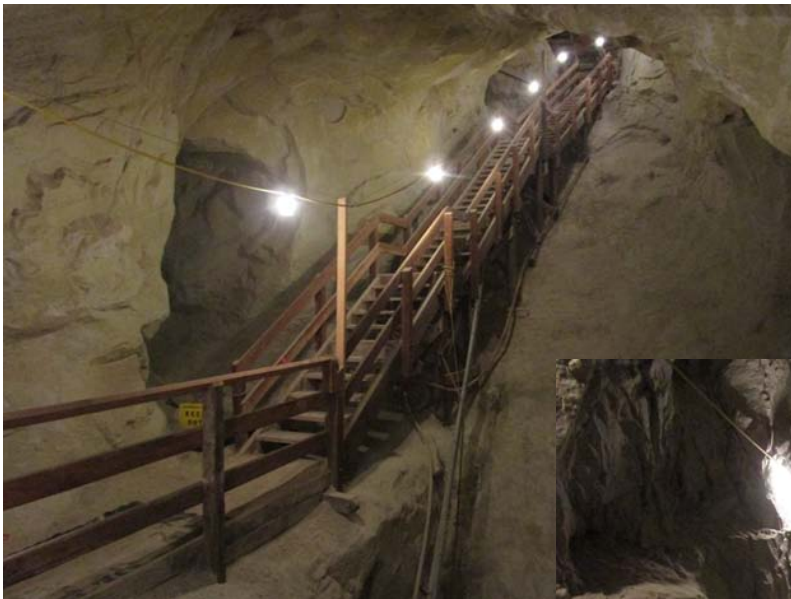
Upward view of stairway.
