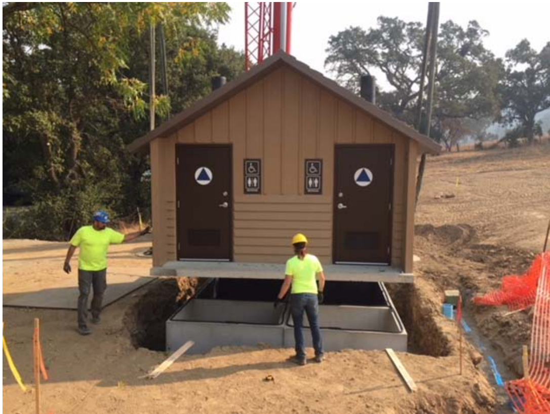
Installation phase of the vault toilet.
