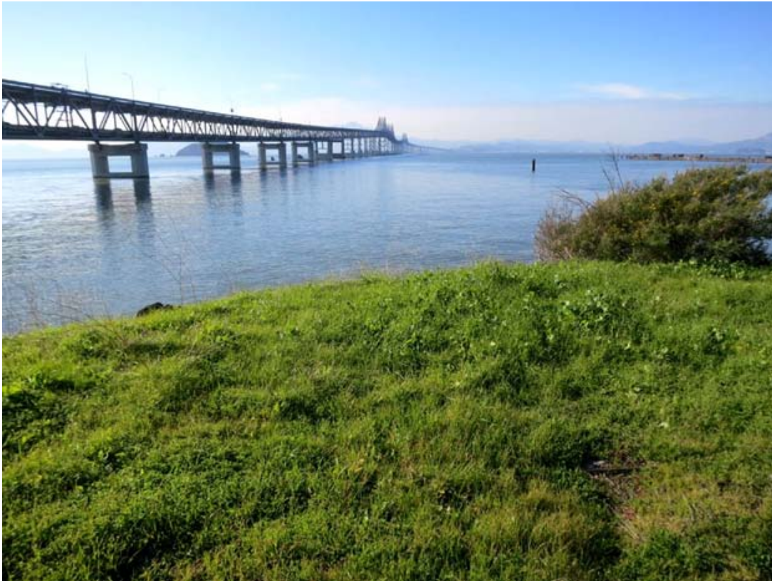
View of Richmond San Rafael Bridge towards Marin from Point Molate.
