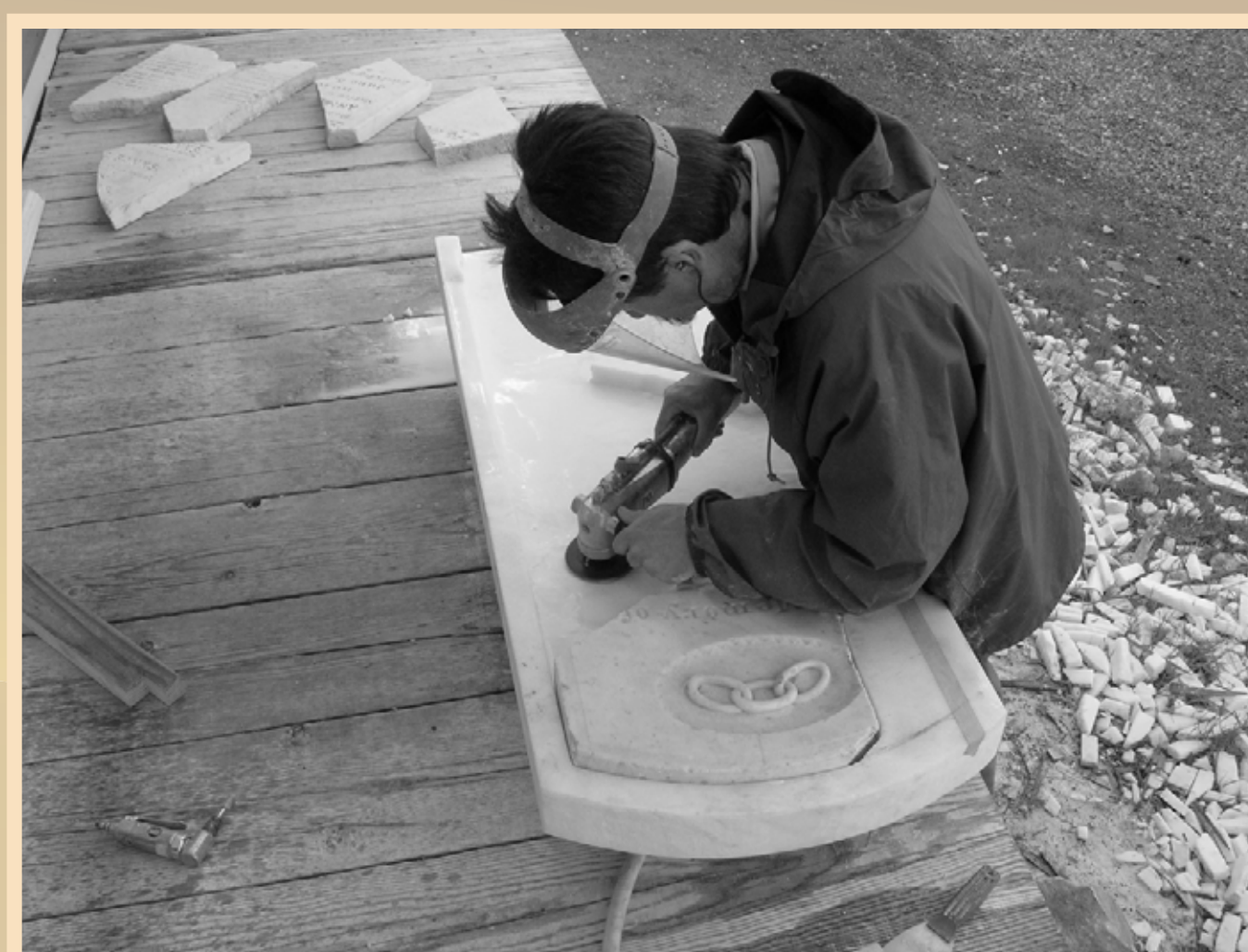
Black Diamond Park Ranger, Doug Fowler, prepares a marble slab to encase the broken pieces of the Joseph Banks gravestone in September 2009.
