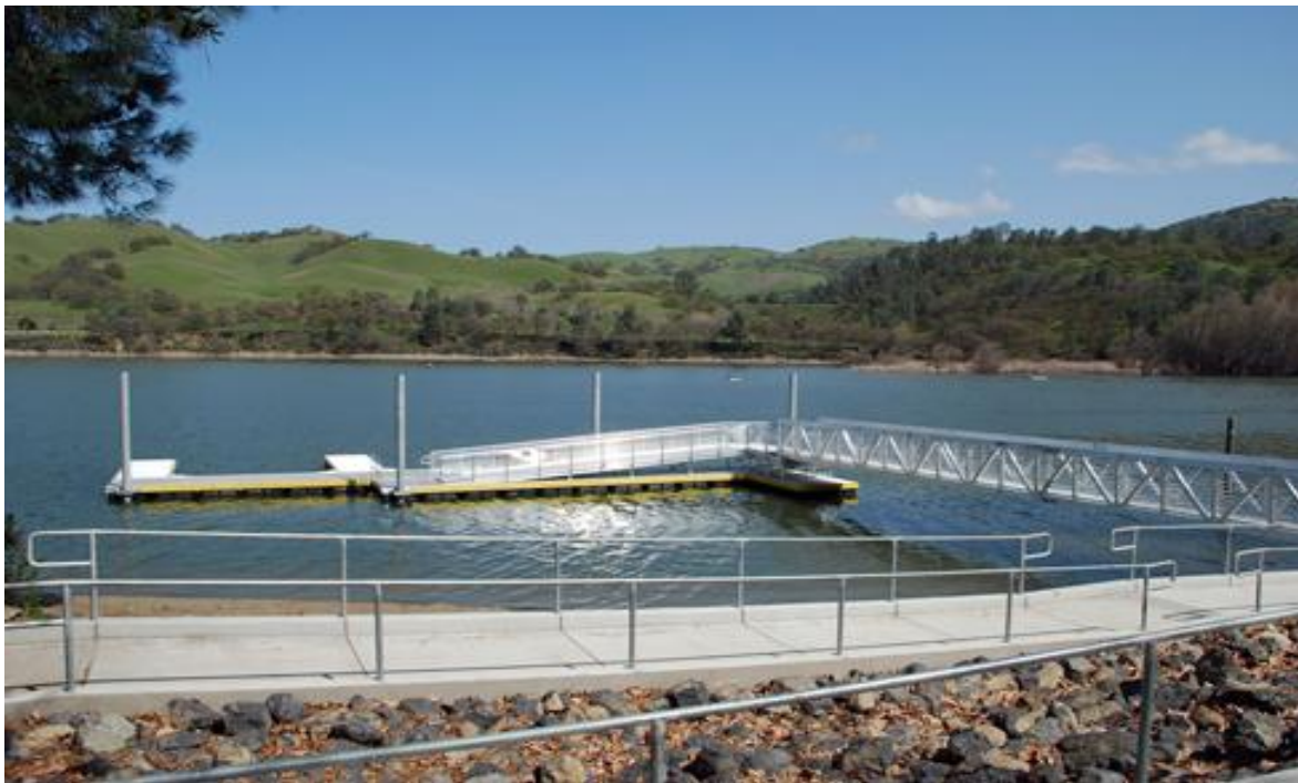
The new fishing and boating dock provides ADA access to Lake Del Valle, the five-mile long centerpiece of the park.
