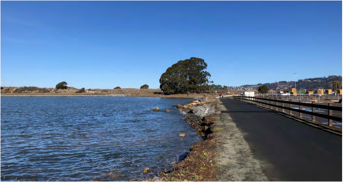
BAY TRAIL INUNDATION NEAR ALBANY BEACH DURING A KING TIDE IN DECEMBER 2020 Source: King Tide California Project
