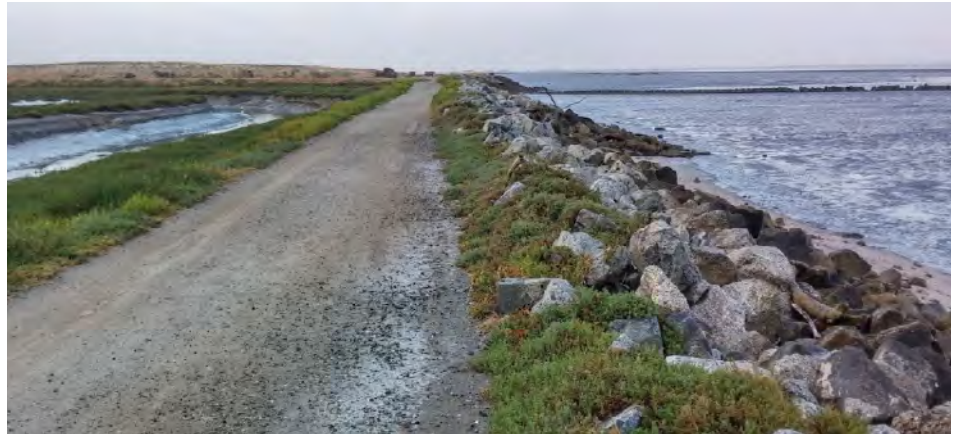
EARTHEN LEVEES AND DIKES - HAYWARD SHORELINE Source: Google Map
