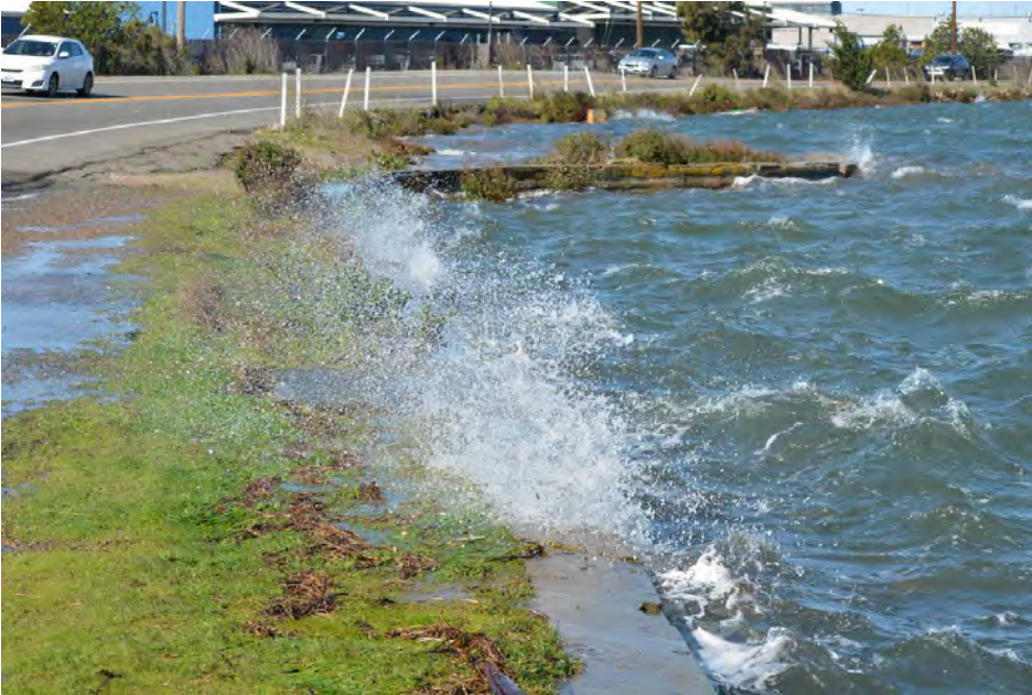
DOOLITTLE DRIVE AT SWAN WAY, OAKLAND Source: King Tide California Project
