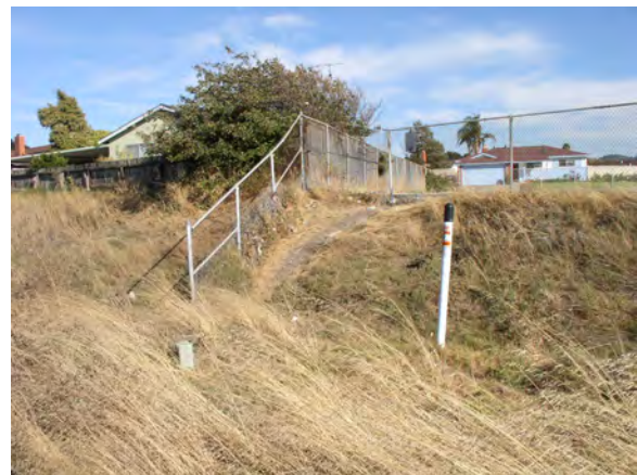
User defined pathways from adjacent properties show a clear pattern of trespassing. This photo illustrates a cut fence and worn trail leading from the Sea View School parking area into the UPRR ROW.
