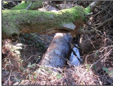
30 Deteriorated culverted channel in proposed Alder Creek restoration area in McCosker sub-area
