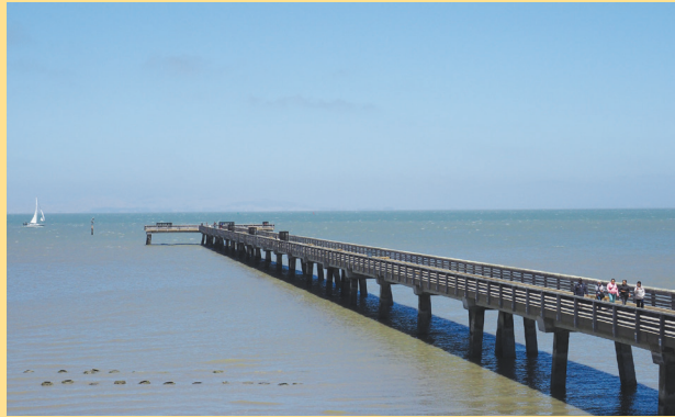
The fishing pier is about 0.6 miles from the Atlas Bridge parking lot. The old pier had a single railroad track on it for loading barges bound for freighters sailing to the Philippines, Central and South America, and Alaska. You can still see the old pilings.
