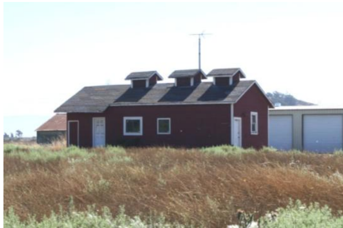
Ardenwood Milk House building
