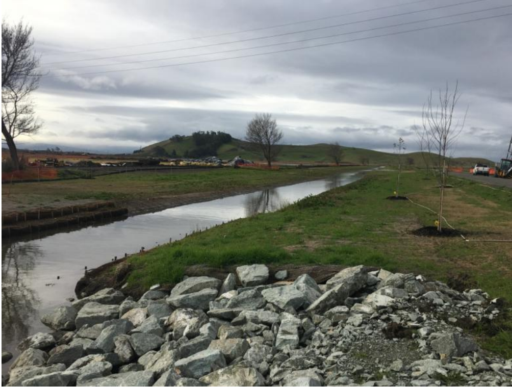
Line P (Ardenwood Creek) Following Flood Control and Riparian Habitat Work
