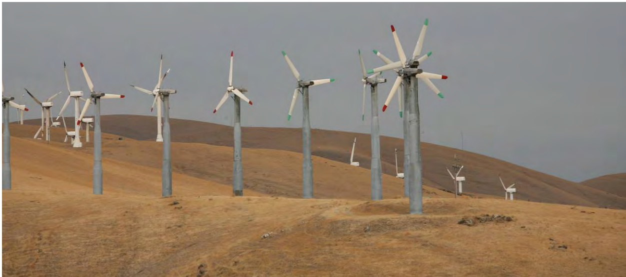
Photo 4. The G string of Nordtank 65-kW wind turbines on the study site, view west-northwest, Souza parcel. Photo by K. S. Smallwood.
