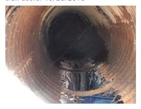
**Photo 10** Near start of Segment B (south end). Existing storm drain outfall proposed for removal and replacement, or daylighting with boardwalk over flow path. 10/26/2015
