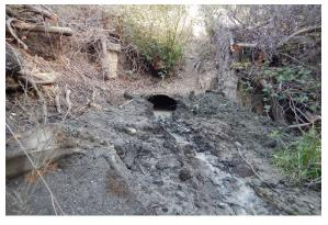
**Photo 9** Near start of Segment B (south end). Clogged storm drain pipe conveying upland and street runoff through proposed trail alignment into Bay via existing outfall. 10/26/2015
