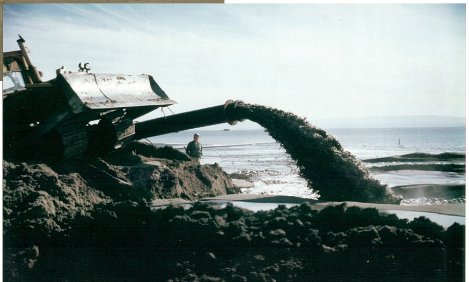
The photo on the right illustrates the process of sand pumped onshore via pipeline in a slurry of sand and water.
