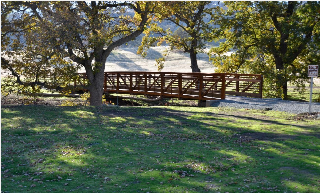
Construction of a pedestrian/bicycle bridge over Round Valley Creek helps control creek erosion and provides opportunity for year round use of a new loop trail connection at this formerly seasonal crossing. (southeast view)
