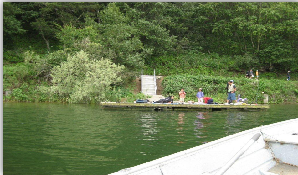
Front view of the stairway leading to the fishing dock.
