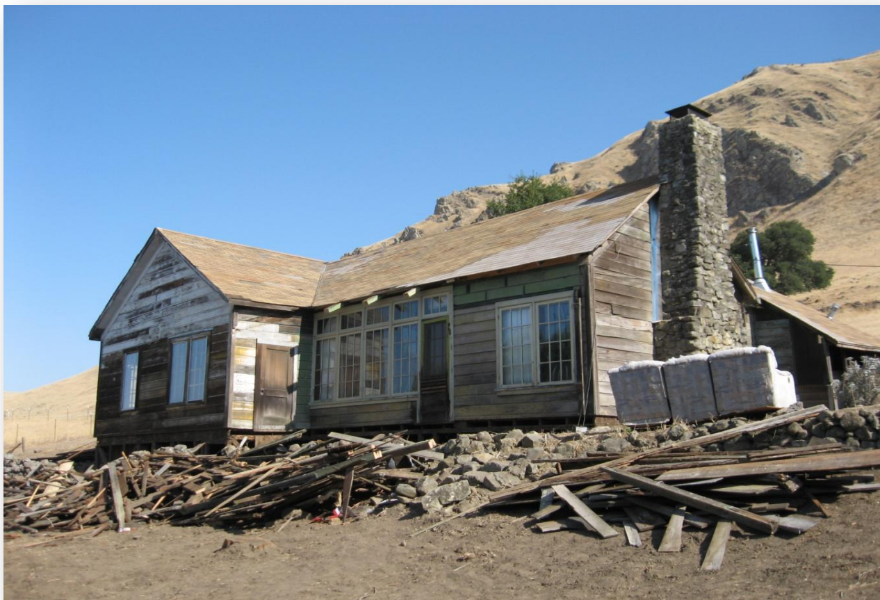
McClure Ranch house before foundation was installed.
