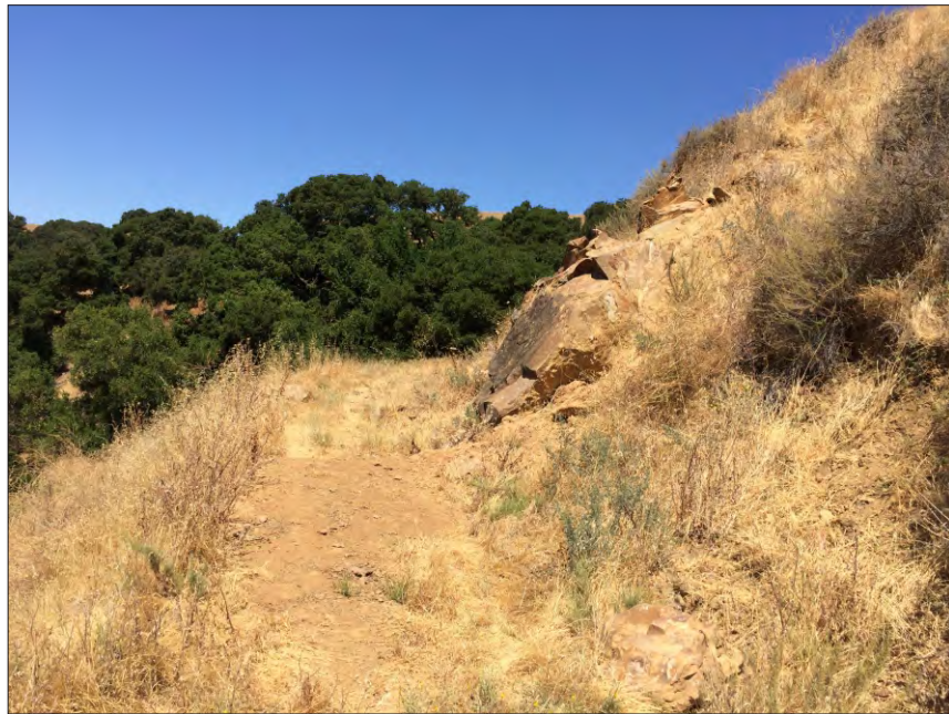
Photo 8 - Landslide damage along trail.
