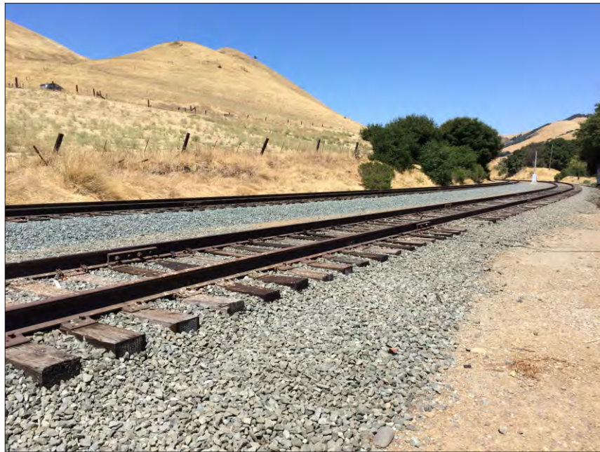
Photo 18 - Railroad crossing location.
