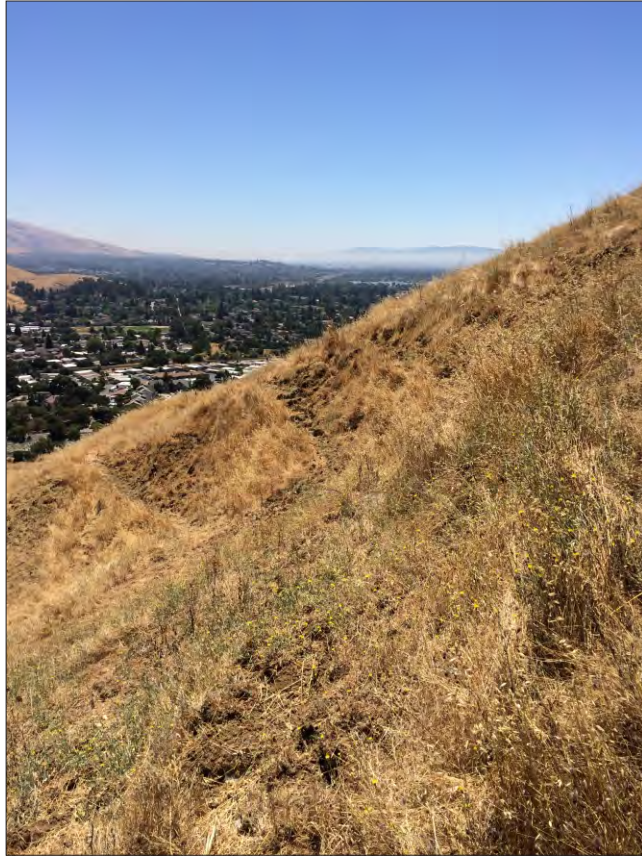
Photo 17 - Existing landslide along trail alignment.
