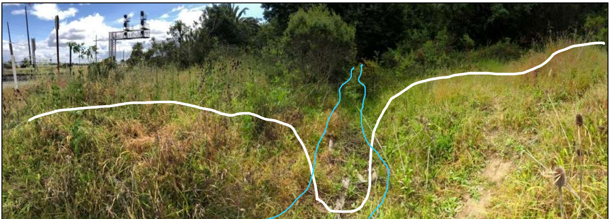
Photo 11. ED-1 as it continues into the ARDA. The markup depicts the topography and channel depth. The channel becomes vegetated in this section.
