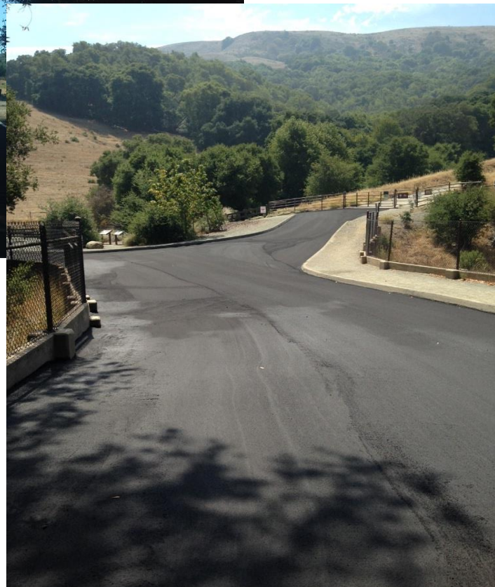
Las Trampas staging area completed.
