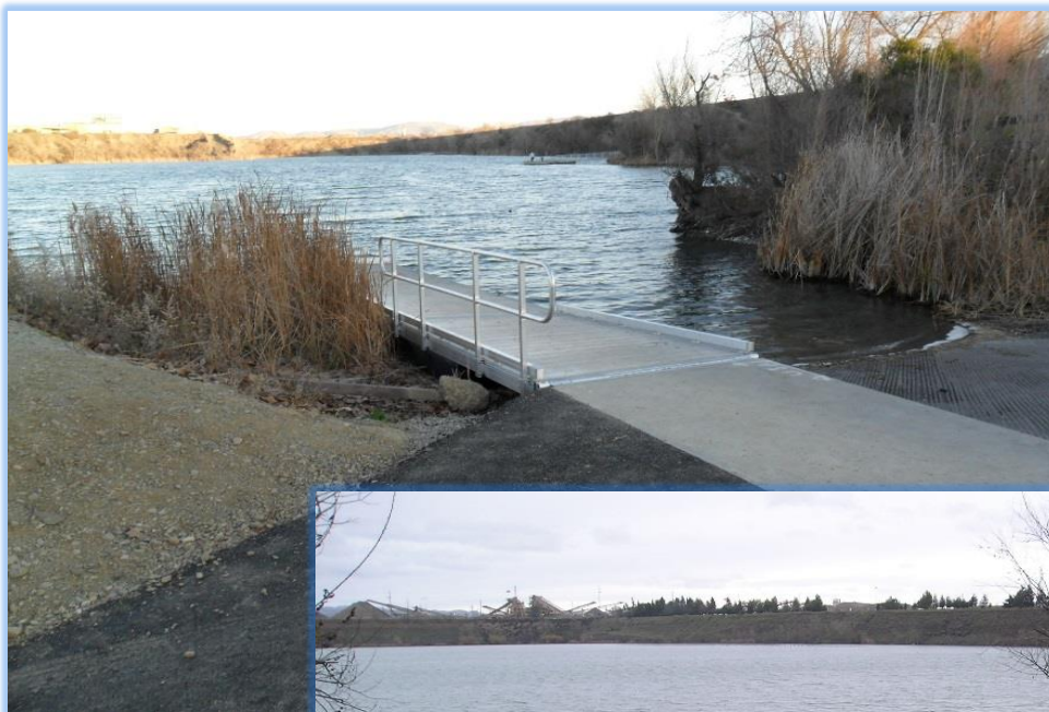
East dock replacement.
