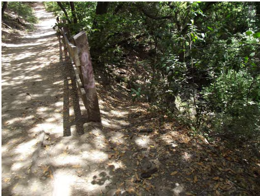
Location 3: 2nd split-rail fence upstream from Nook Pool. This steep trail appears to be caused by water erosion. Fencing should be extended to discourage animals or people from entering. A retaining wall could prevent further erosion.
