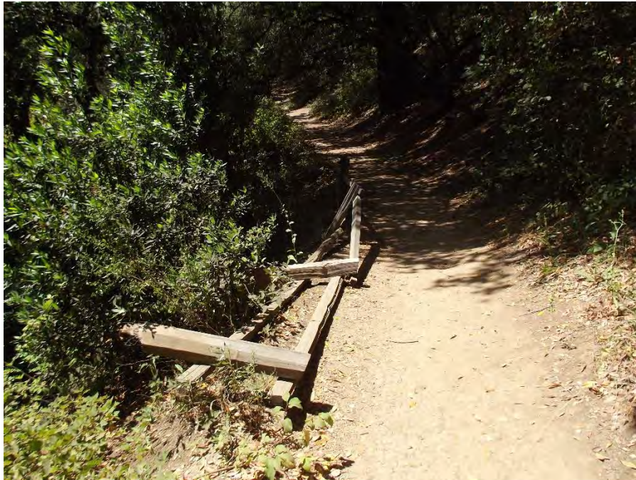
Location 4: Upstream from site 3. Fence in need of repair.
