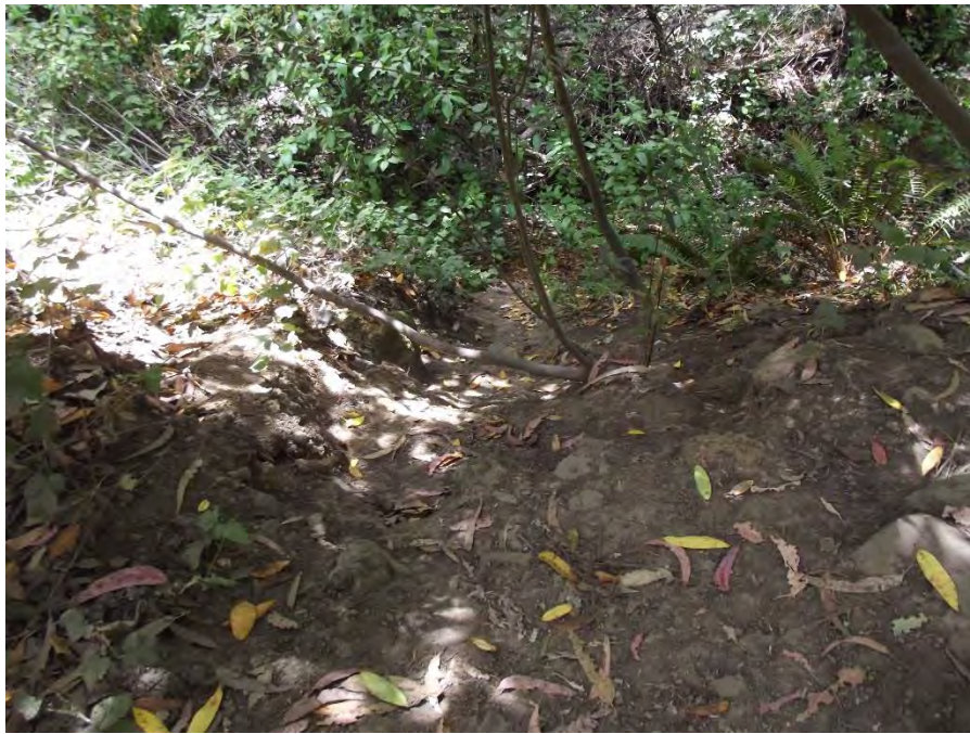
Location 15: Upstream from redwood fence. Erosion is evident but it is uncertain how it was caused. A fence should be erected to deter hikers and animals from entering.
