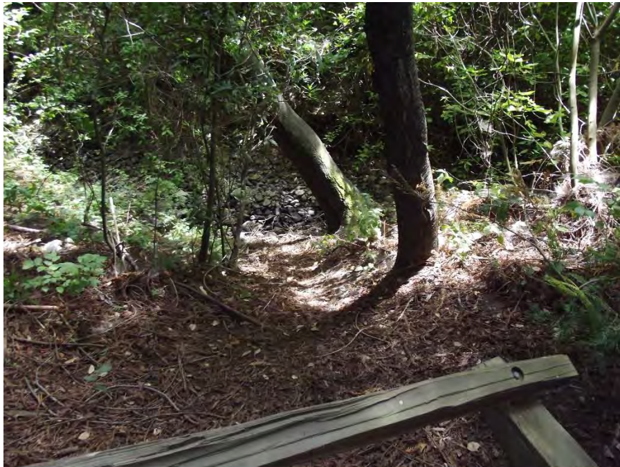
Location 6: Redwood grove. Fencing is falling over and in need of repair. Bootleg trail is very close to creek—a very easy access point for people and dogs.
