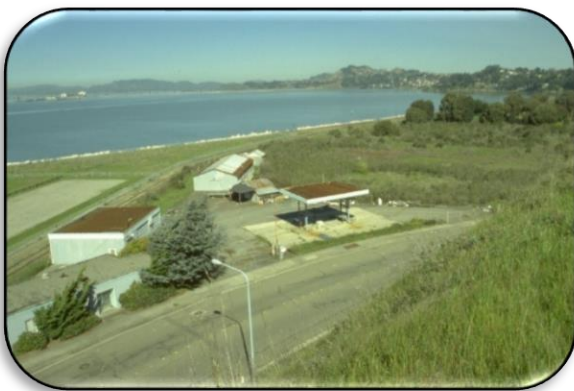
Bray property before structures were removed District archives. Photographer unknown.
