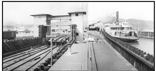
Ferry Point pier, circa 1915. Ferryboat San Pablo in foreground, the Ocean Wave is in the background. Photo also shows a freight barge on the left, the gallows structure, dolphin piles and apron of the freight/car float slip.
