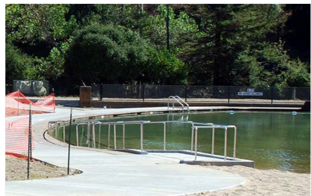
Improvements to the Lagoon (top, left) include a new water distribution system (top, right) and a re-contoured, resurfaced floor (above, left). The new ADA-accessible ramp is shown (above, right). The rehabilitation of the Don Castro Lagoon focused on improving water quality by installing new filtration and sanitation equipment as well as on providing ADA-compliant access to this popular swimming venue.
