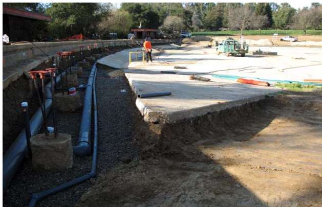
Improvements to the Lagoon (top, left) include a new water distribution system (top, right) and a re-contoured, resurfaced floor (above, left). The new ADA-accessible ramp is shown (above, right). The rehabilitation of the Don Castro Lagoon focused on improving water quality by installing new filtration and sanitation equipment as well as on providing ADA-compliant access to this popular swimming venue.
