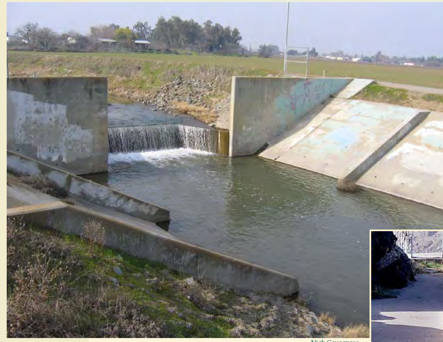
Concrete drop-structure on Marsh Creek
