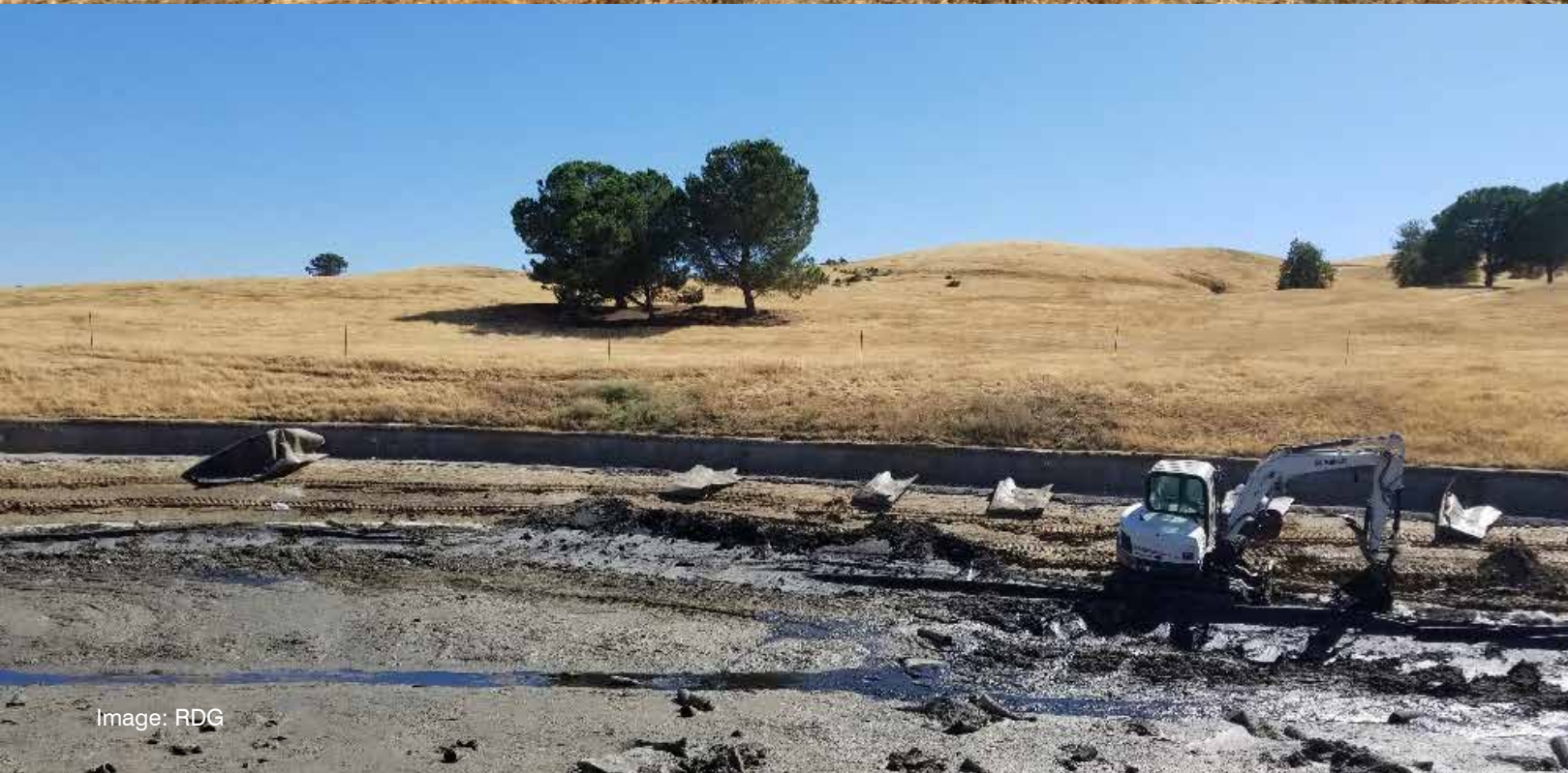
Construction crews dig test pits (top) and remove the pond liners at the former Roddy Ranch Golf Course.
